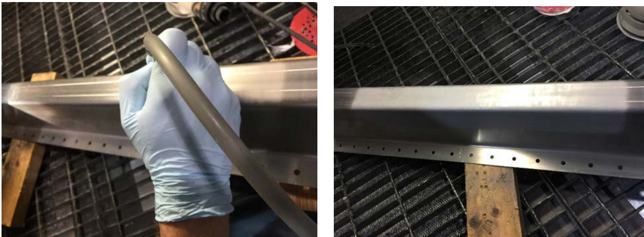
Figure 7-25. Surface Preparation of Steel Rocker
