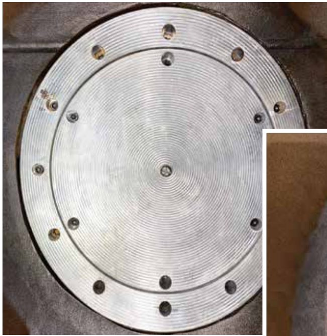
Design engineered prefabricated metal plug installed to cover a 20-inch lateral and provide bearing surface for liner inversion
