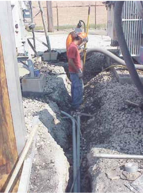
A major growth opportunity for vacuum excavation is in the electric utility market
