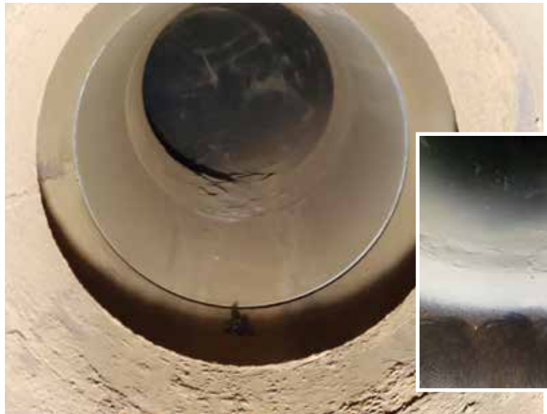
Use of aggregate and mastic epoxy to bridge 30-inch valve gate well was done for the first time ever
