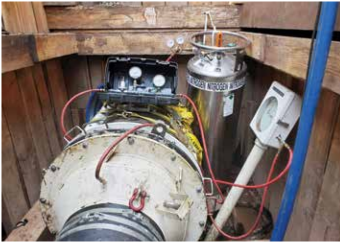
Liner ambient cured with nitrogen supplied as make-up air
