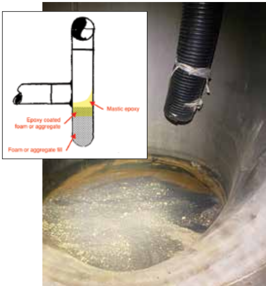
Stack was backfilled, then covered with mastic epoxy to form a 90-degree elbow from the 36x36-inch Tee
