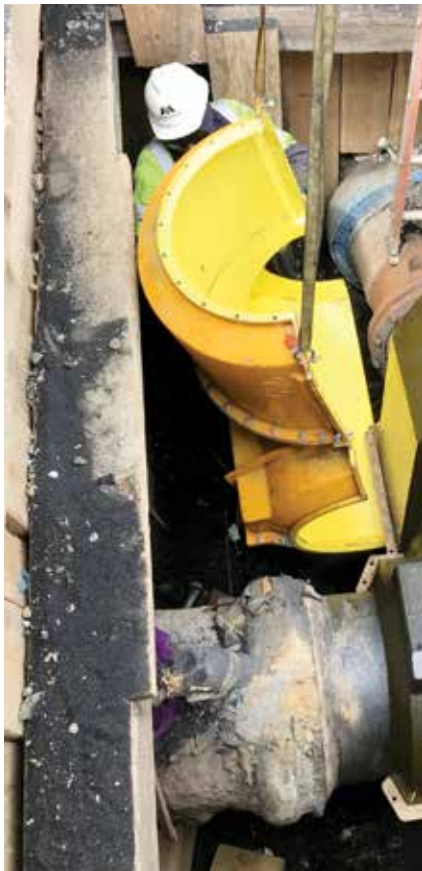
A custom-made mold is lowered into the excavation before being installed onto the leaking fitting
