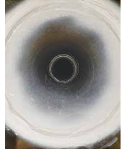
Application of high-strength heated epoxy spray to reinforce and seal leading 36x30-inch reducer was a breakthrough technical accomplishment
