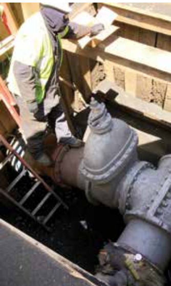
After descaling and sandblasting, the fitting is ready for primer
