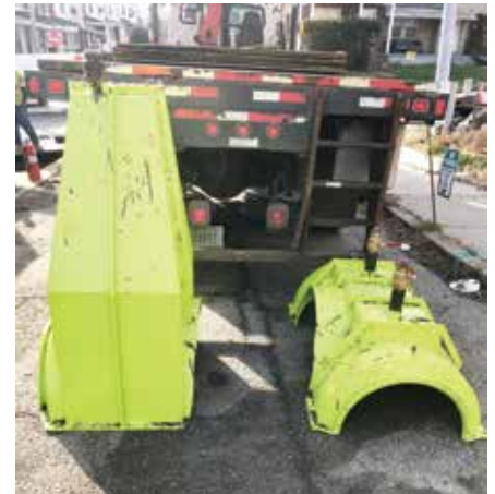
A steel mold, custom made at the Miller Pipeline fabrication shop in Indianapolis, after the leak has been repaired
