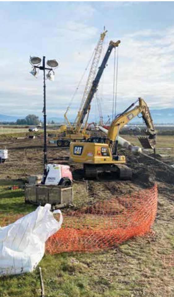
Figure 1. Maxi-Sized HDD Installation
