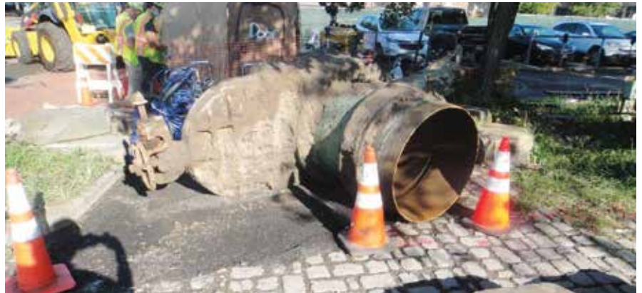
36-inch Valve was excavated on the east side of the “The Mess” to form the Receiving Pit for liner inversion
