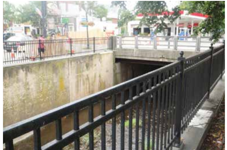
Pipe configuration of "The Mess" was built in 1971 when the Rahway River in South Orange NJ was encased in a concrete channel and the bridge widened
