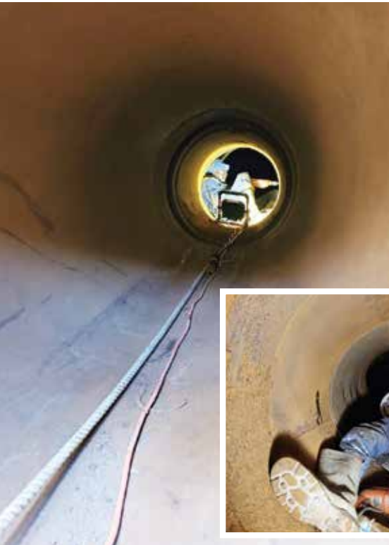
Injected curtain grouting into the surrounding soil from the interior of the pipe was again used to prevent water entry into the depressurized main
