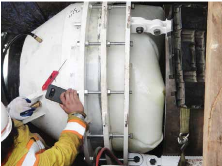
36-inch Guide Pipe was essential to ensure 36-inch liner was aligned correctly as it traveled through the 30-inch segment
