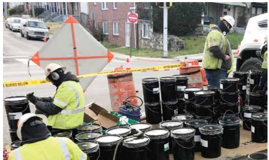
The crew preps the Encapsal resin for pouring
