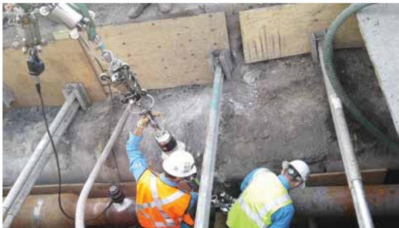
Figure 3. Deployment from a compact urban bell hole for a California utility
