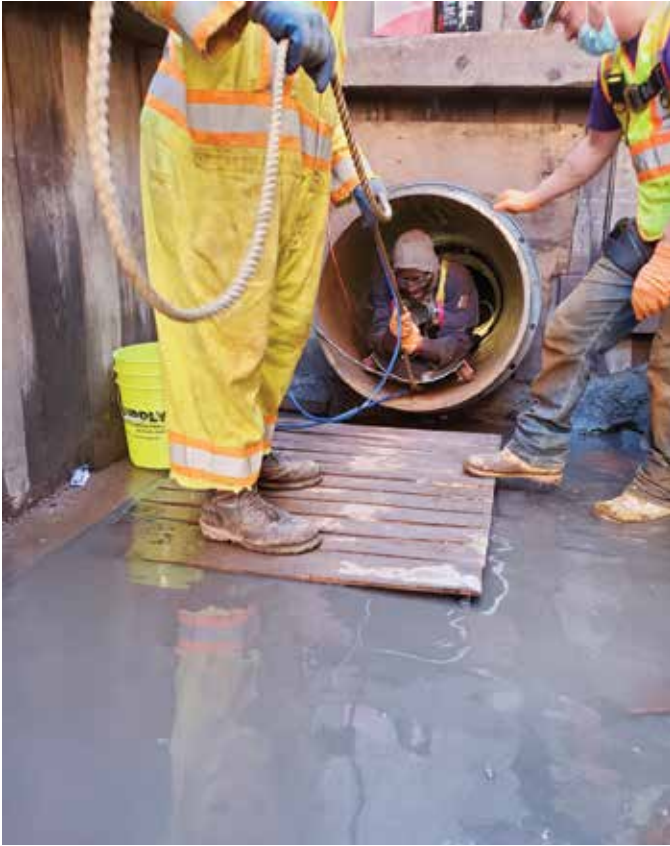
Confined space entry with extensive safety precautions was necessary for several preparatory steps prior to lining
