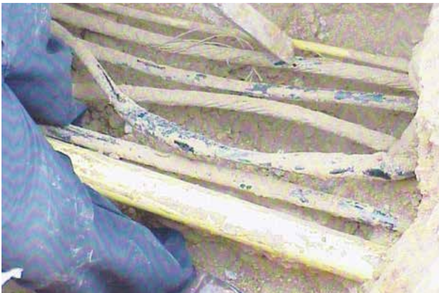
Older buried electrical lines are subject to insulation breakdowns
