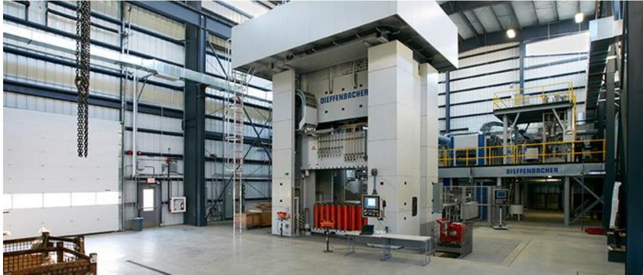
Figure II.2.3.17. The Fraunhofer facility. Source: Fraunhofer Project Center.
