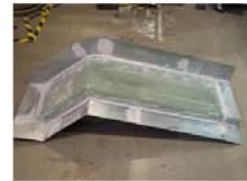
Fill crevices and build corner fillets.
